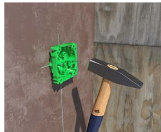
Fixing by means of steel nails.
