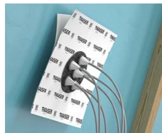
...glue the sleeve in position and thoroughly smooth it onto the surface, working from the inside to the outside.
