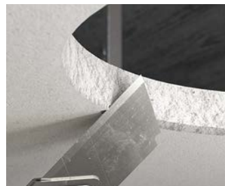
Chamfer the installation opening for mounting flush with the ceiling or wall using a cutter knife.
