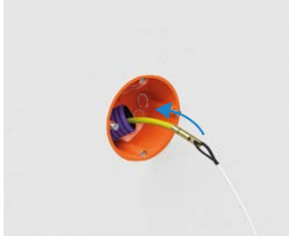
Connect the pull-in aid to the cable end and pull it into the empty duct.
