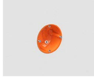
One-gang box installed with micro duct.
