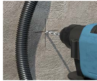
Cut \varnothing 8 mm drill hole at least 50 mm deep.
