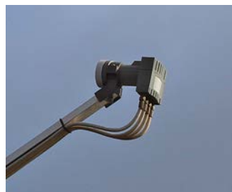
4 coaxial cables are connected here for reception.
