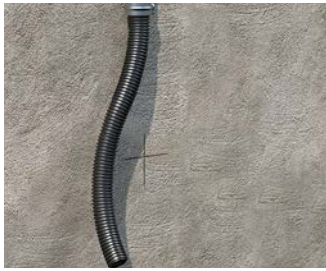
Masonry with conduit exit.
