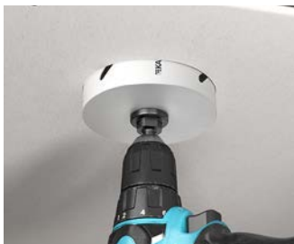
Cut installation opening Ø 120 mm with KAISER BASIC cutter (Art. No. 1084-20).
