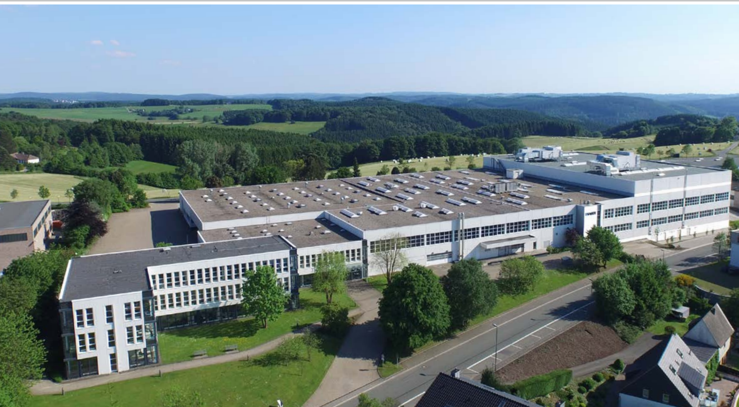
KAISER headquarters Schalksmühle, Germany
