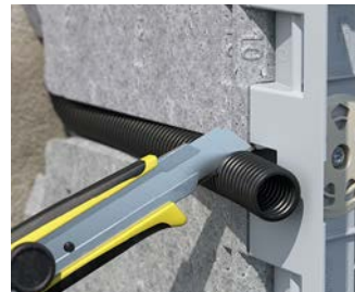
Press the conduit into the sidewall guide and cut it to length.
