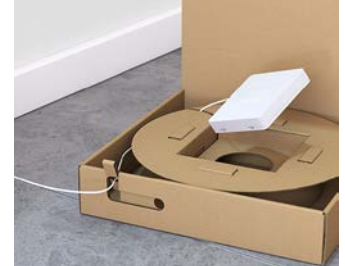
At the end, remove the optical termination outlet from the cardboard box and pull in the remaining cable.
