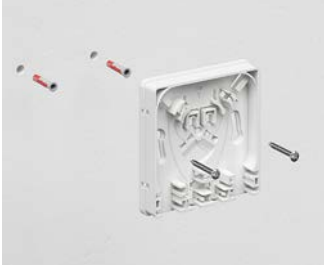
Make 5 mm drill holes.
