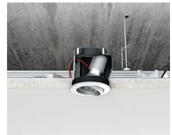
...and installing plasterboard.
