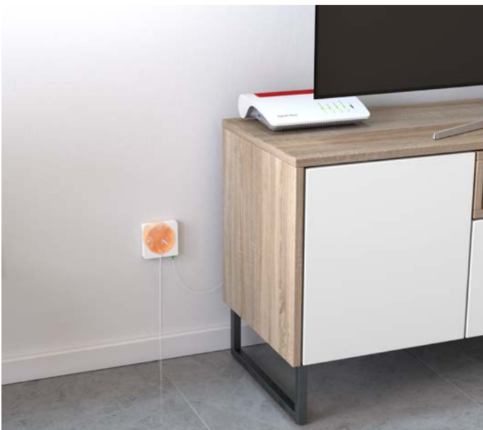
Now mount the optical termination outlet exactly on the device box, wall or multimedia panel.
