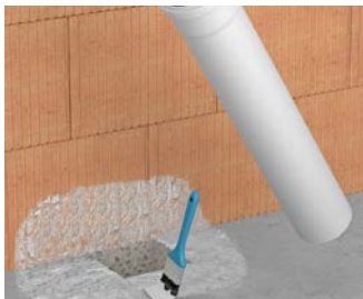
Pre-treat mineral bases and fibreboards with primer.
