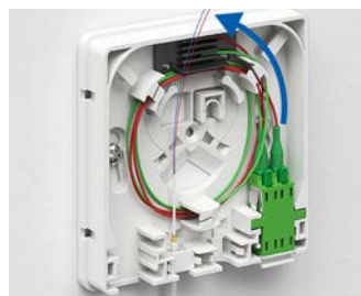
Insert, guide and put pigtails in place.
