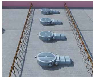
Prefabricated element with integrated HaloX® housings is laid on concrete building site.
