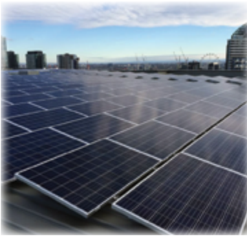
Southern mounting type tin rooftop
