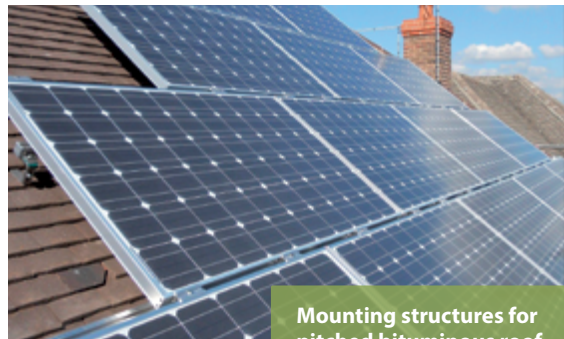
Mounting structures for pitched tiled roof
