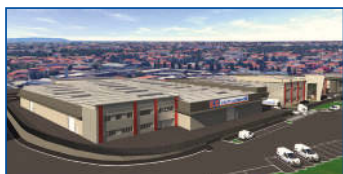
NEW PRODUCTION FACILITIES 2019 Scanzorosciate (BG)
